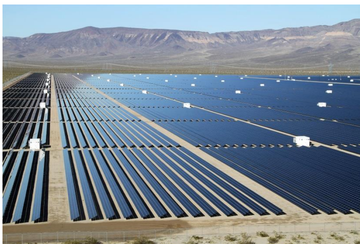
Sempra U.S. Gas and Power received a GOE tax incentive for the Copper Mountain Solar II, III, and IV power plants in Clark County, NV.
